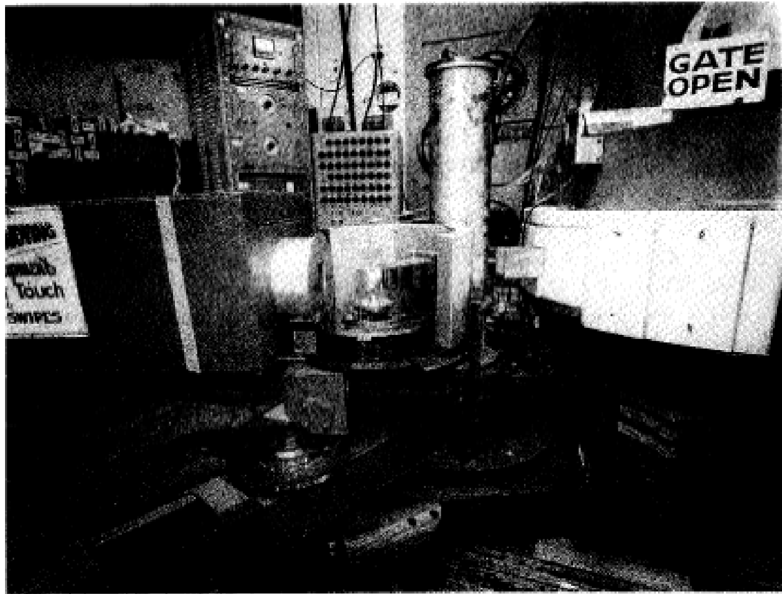
Fig. 9: Photograph (1959) of the original triple-axis spectrometer at the NRU reactor at Chalk River. The bank of 52 rotary switches, preset to go through an energy scan of up to 26 points, can be seen in the upper-centre. One of the three variables involved would traverse linearly through the domain of settings desired, while the other two advance nonlinearly according to the settings of the appropriate switches. (AECL photo)
